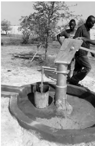
Reverend Aaron dug a new well for Chisomo street children centre.
